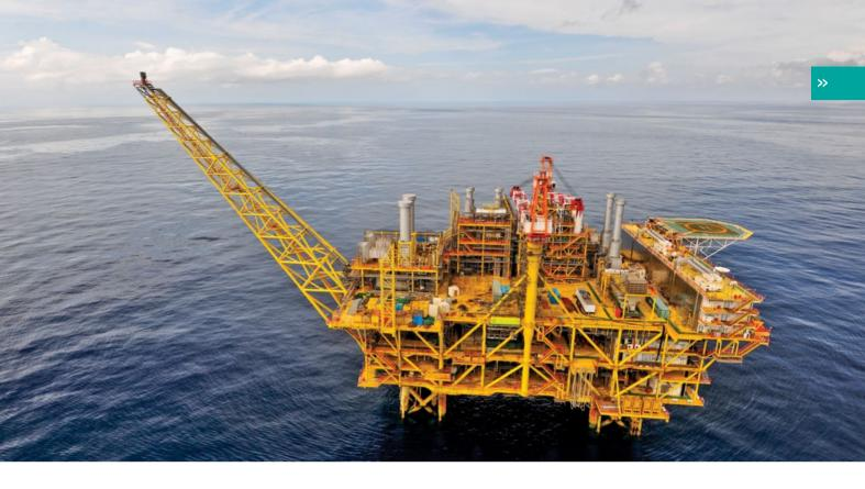
pipes to the onshore processing plant in Zhuhai. Engineers claim this is economic as a single platform can process the output from several nearby oil/gas fields, reducing the amount of deep-sea piping needed to transport output to the onshore gas processing plant.
