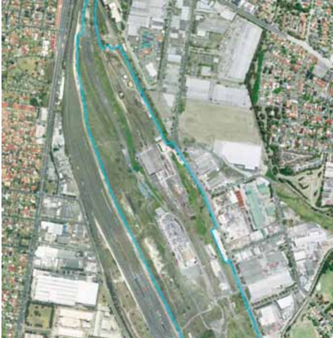
Enfield Intermodal Logistics Centre ( Sydney )
